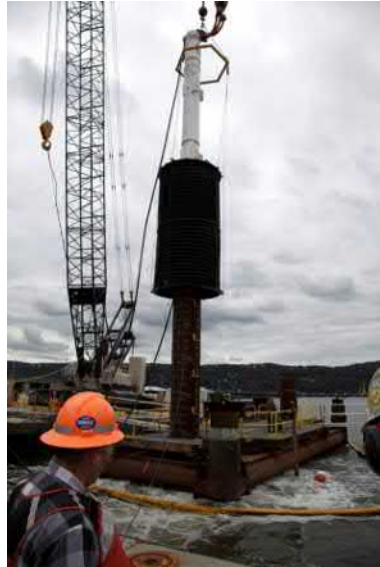
Photo credit: New York State Thruway Authority
