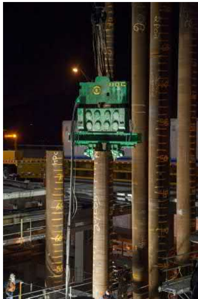
Photo credit: New York State Thruway Authority
